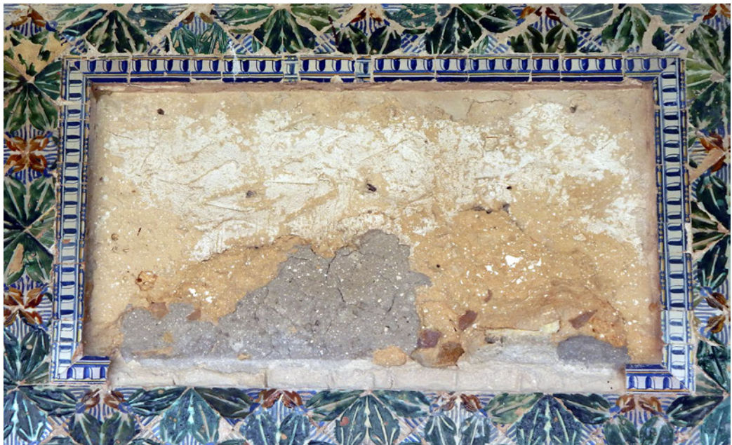
Figure 3. The hollow of the lost Noronha Coat of Arms panel with part of its marginal frame still in place stands against a background of Bacalhôa pattern Hispano-Moresque tiles (image © Associação de Colecções | The Berardo Collection).
